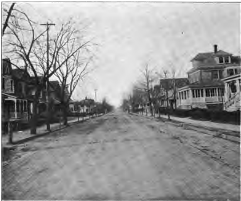
Corliss Avenue, Monmouth Co., after improvement.
